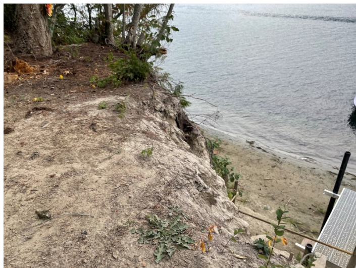
Ricco Property: View from the top of the bank looking waterward
