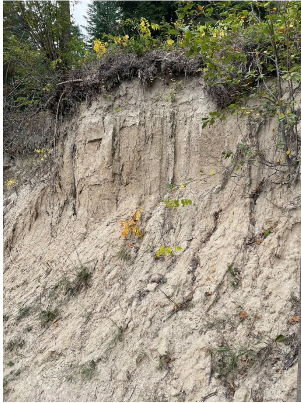
Ricco Property: Mass failure
